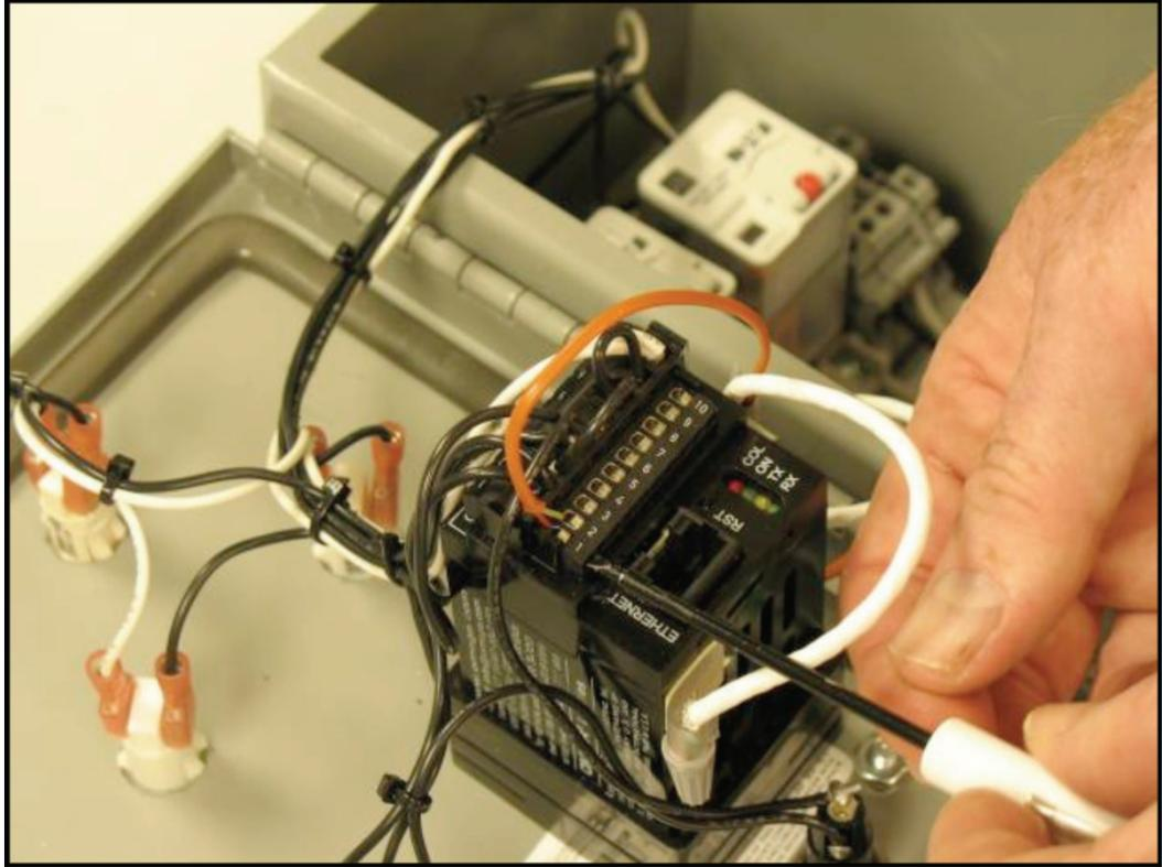
Figure 3-2. Remove The Thermocouple Wire From 1 and 2
