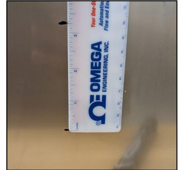
Figure 2: Measure out mounting stud points at 3.5"
