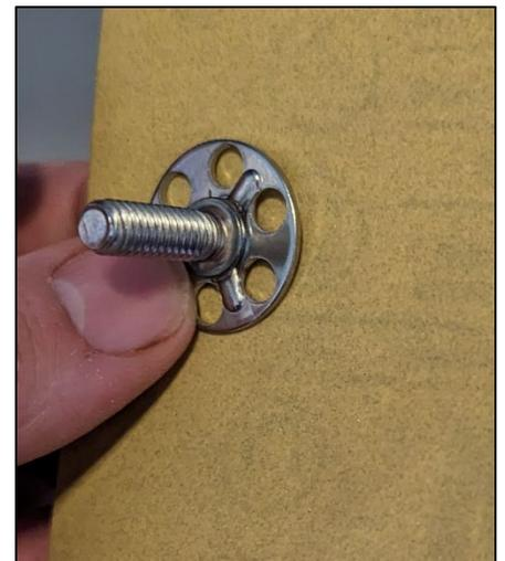
Figure 7: Sand the adhesive studs
