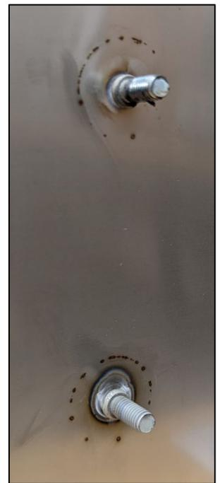
Figure 3: Included studs welded to tank
