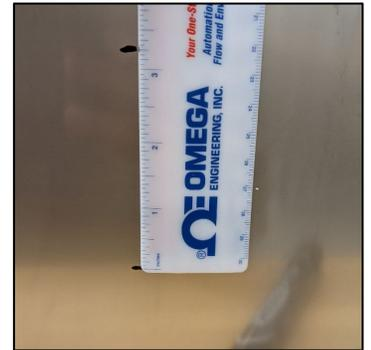
Figure 5: Measure out mounting stud points at 3.5"
